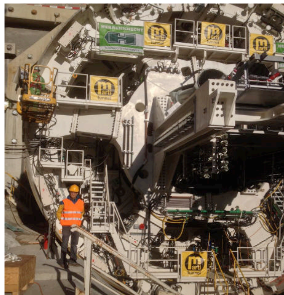
TBM Belchentunnel, Nov 15
